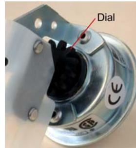
Pressure Switch inside the Enclosure
